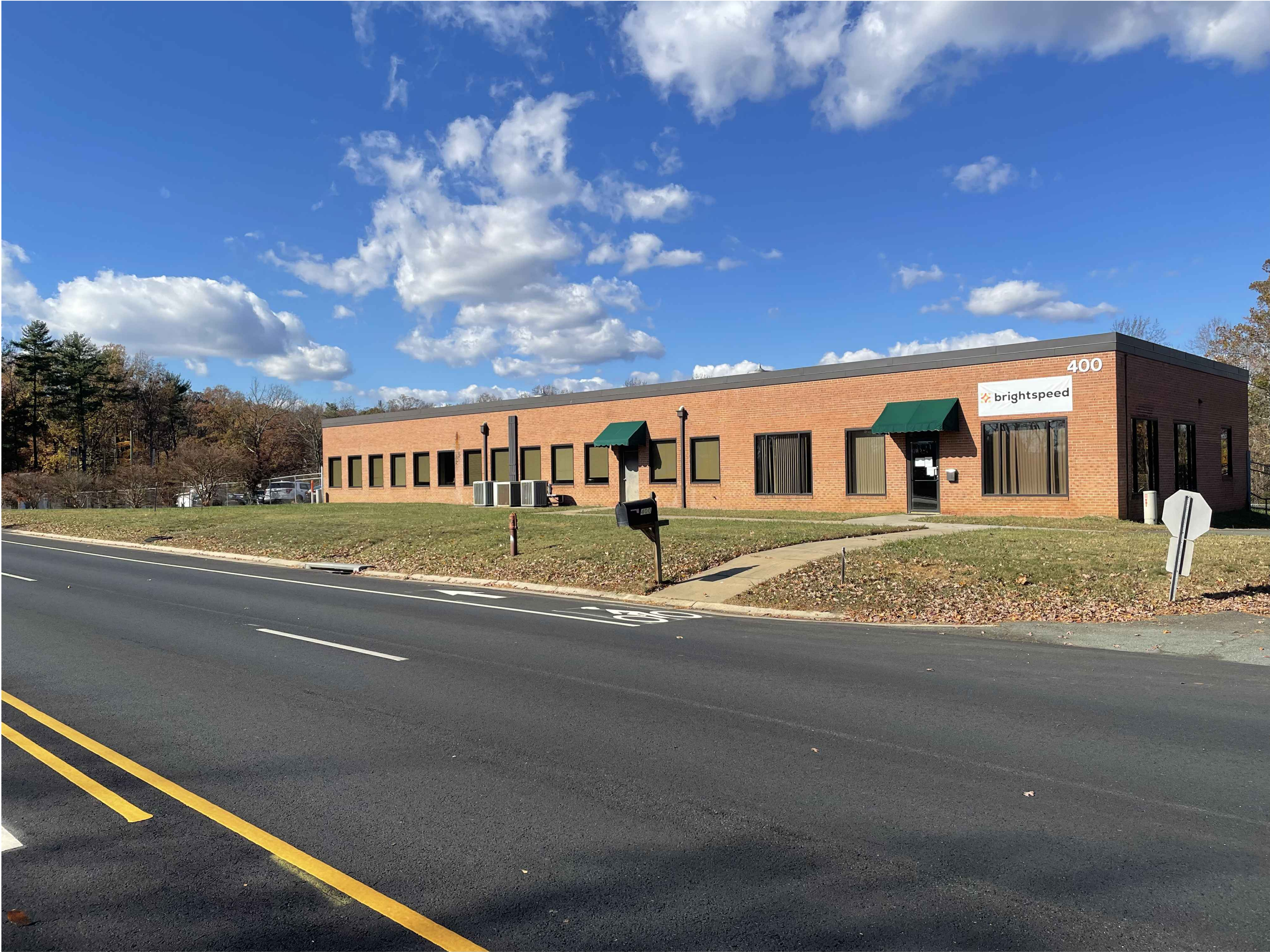
EXISTING FRONTAGE CONDITION - EAST ENTRANCE VIEW
