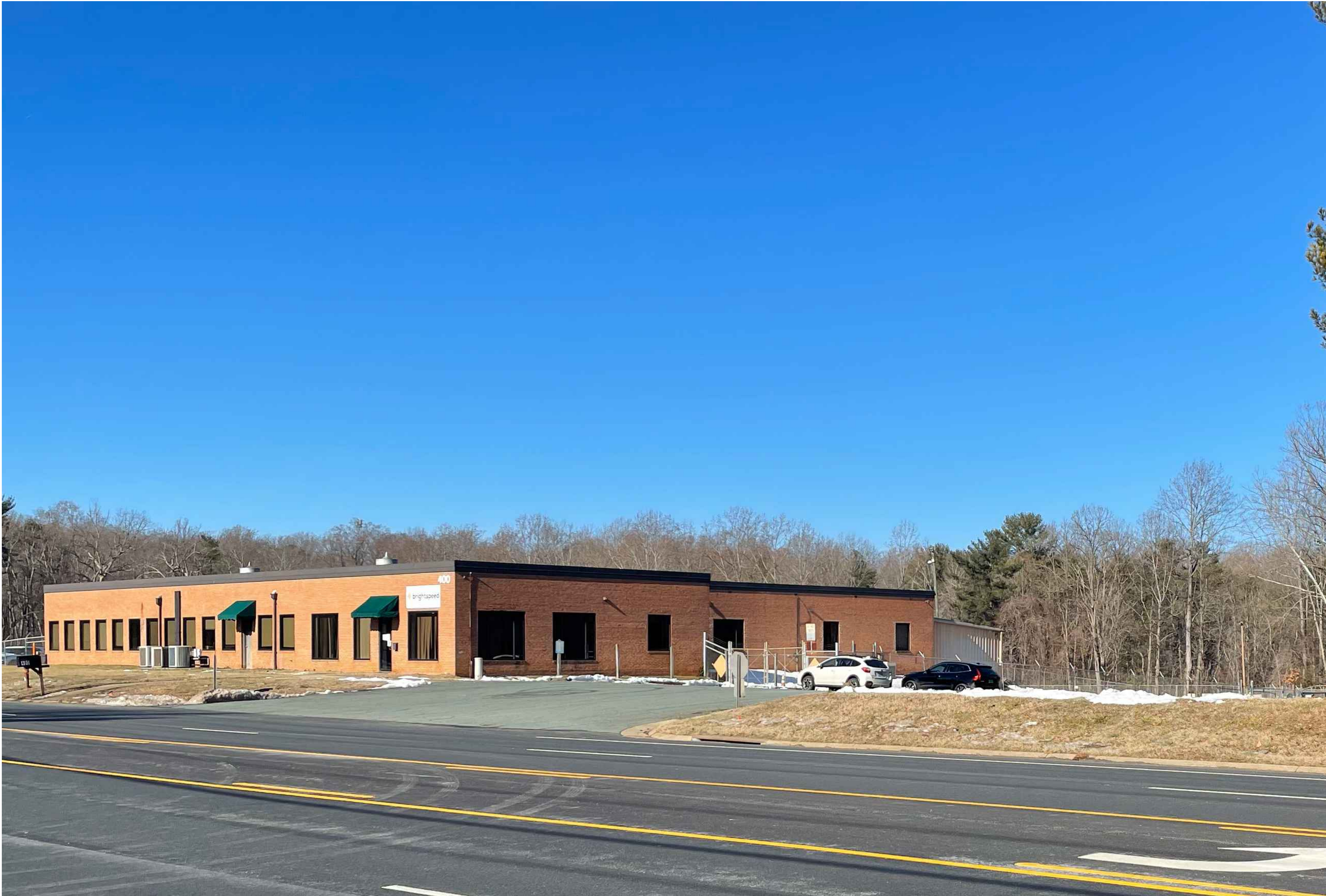
EXISTING FRONTAGE CONDITION - CONTINUED EAST ENTRANCE VIEW
